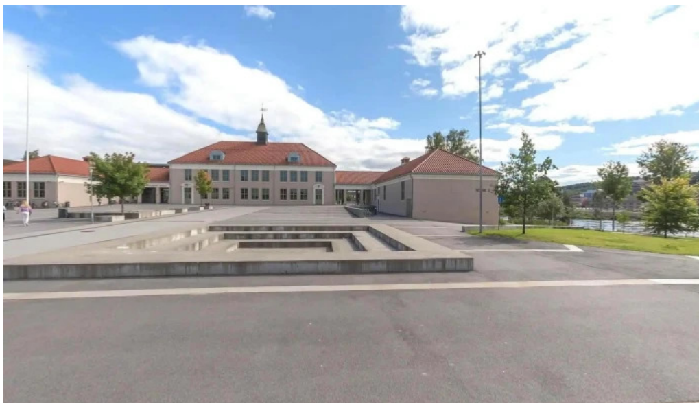
Sentrum videregående skole street view 360deg
