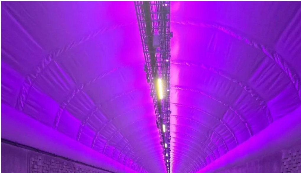
Sykkeltunnel worlds longest bicycle tunnel katalog
