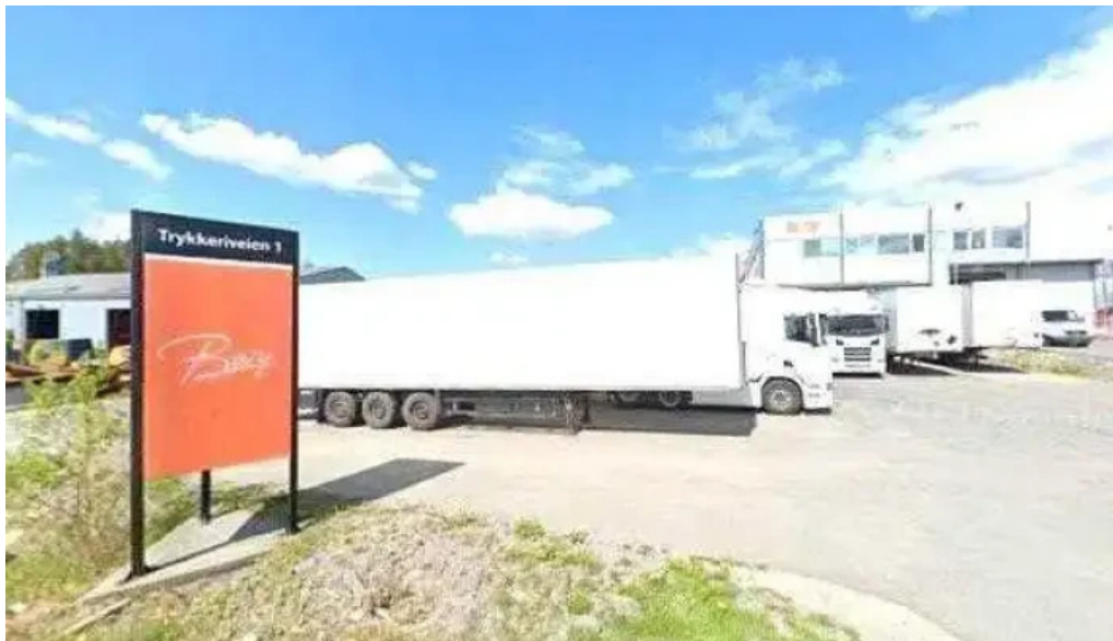
Stack infrastructure osl03 data center campus street view 360deg
