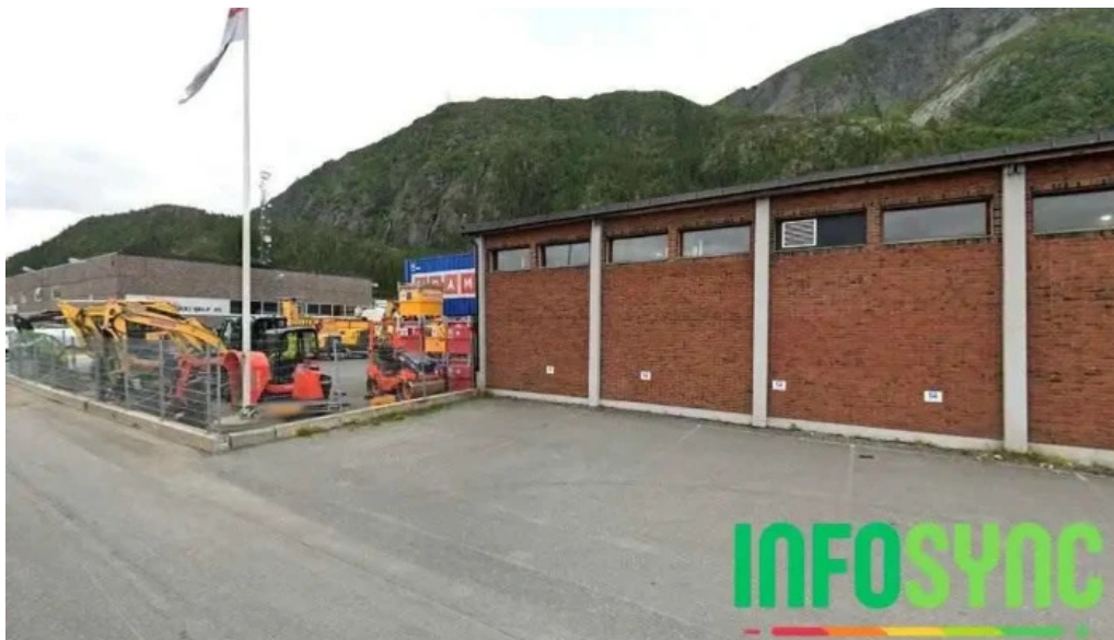
Nye nordland tak as mosjøen
