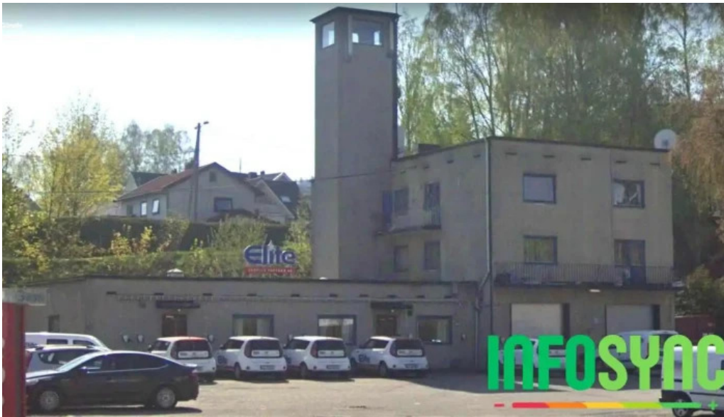
Insider facility solutions as avd drammen drammen
