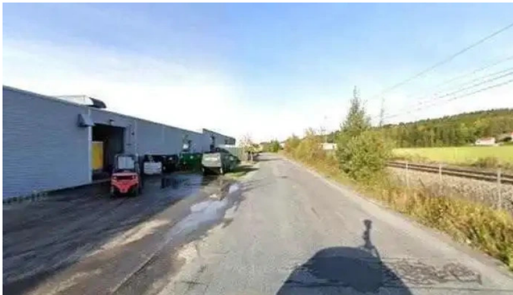
Wican regnskap halden as street view 360deg
