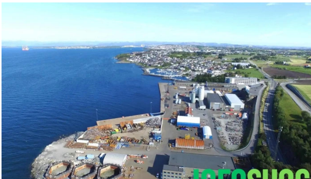
Randaberg coating alle
