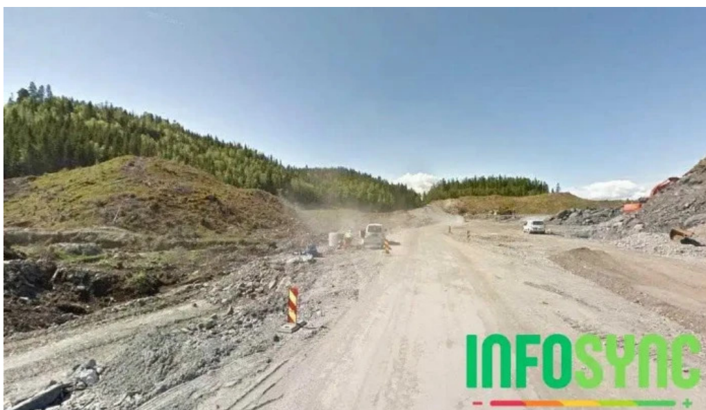
Trøndelag isolering as malvik
