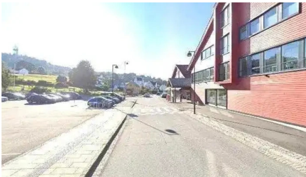
Ups access point street view 360deg
