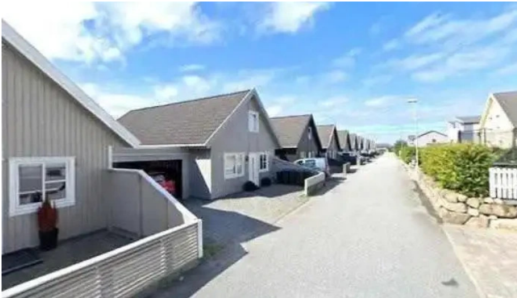
Fjell vandring as street view 360deg
