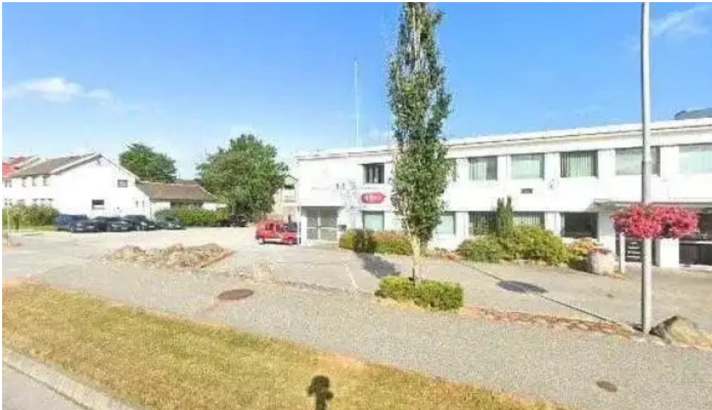
Klepp energi street view 360deg
