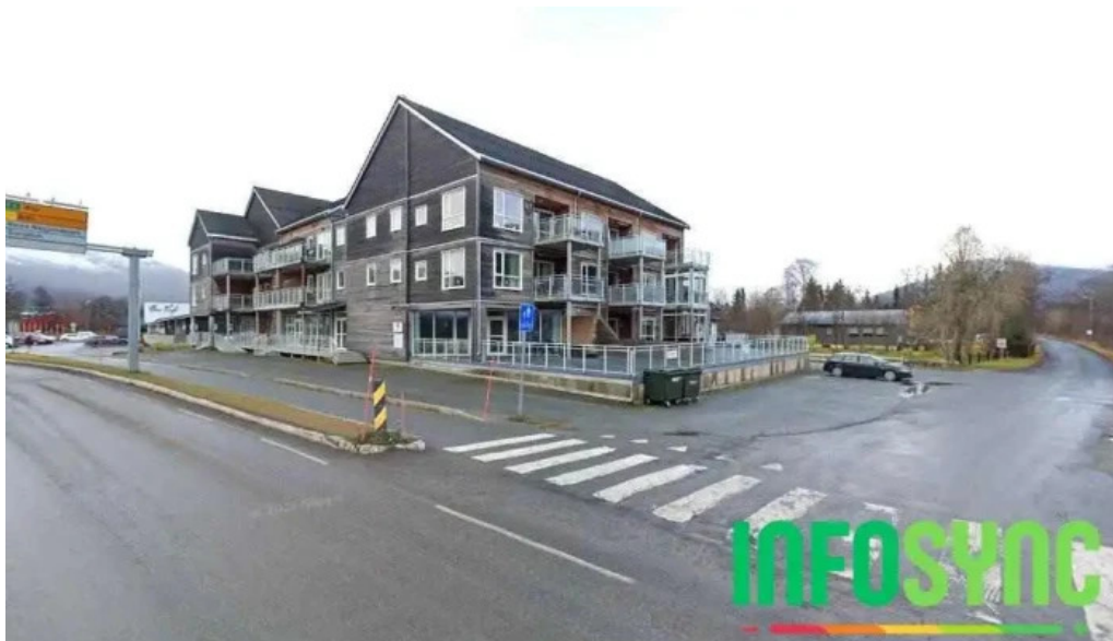
Nord troms skadesanering as storslett
