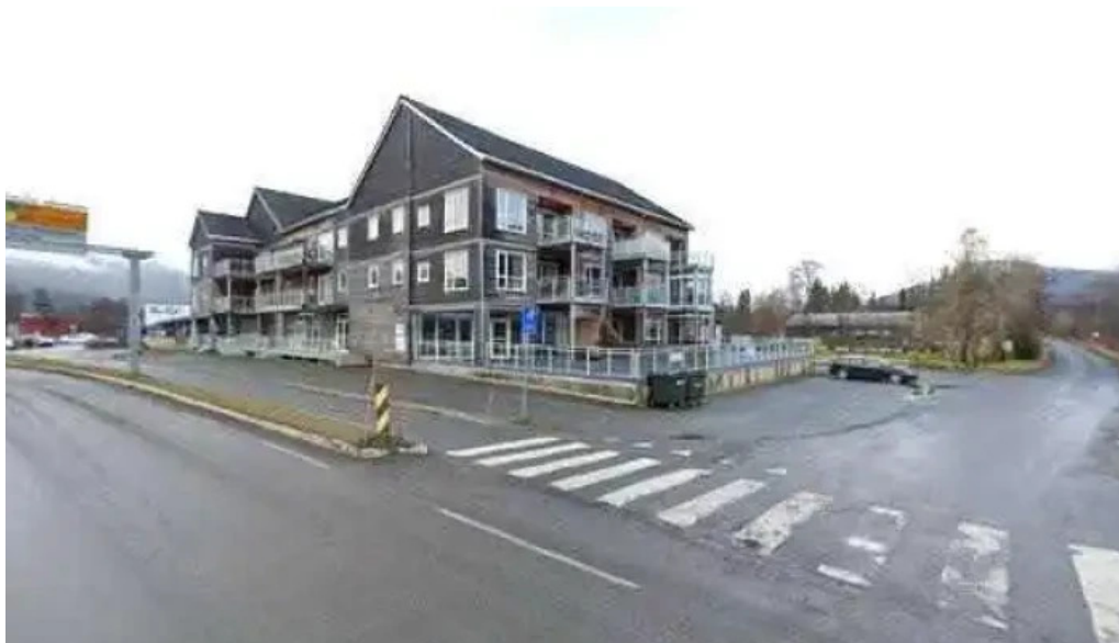
Nord troms skadesanering as alle
