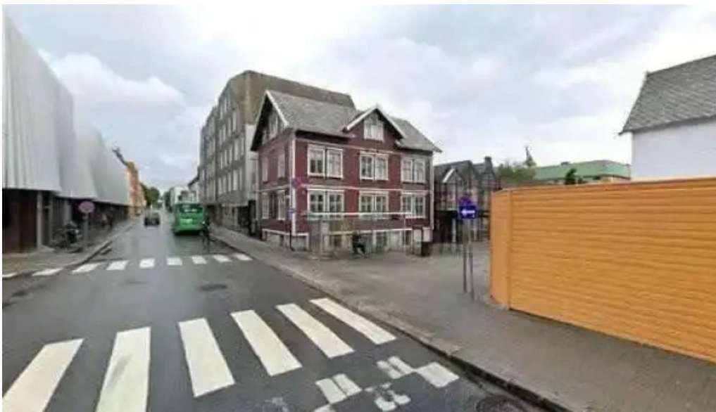
Haugesund medisinske senter street view 360deg
